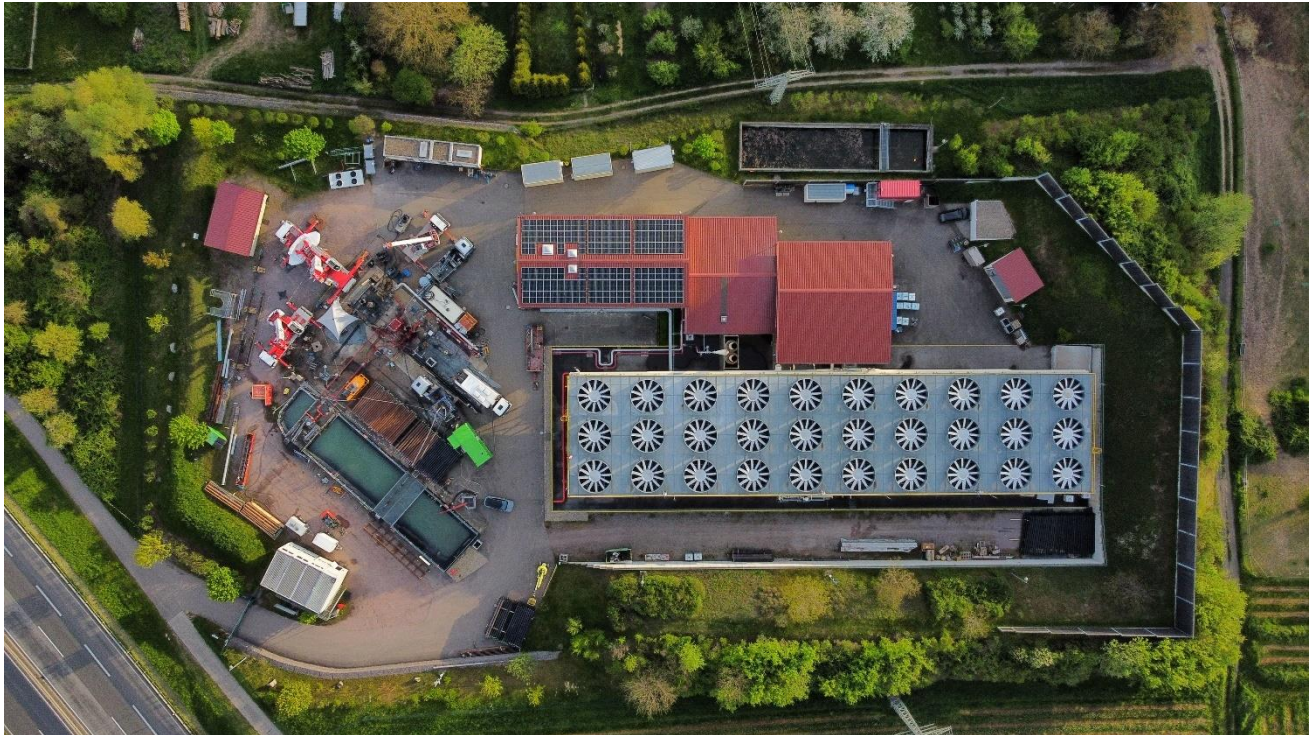
Figure 7 Aerial photograph of Vulcan's Natürliche Insheim Geothermal Plant.
