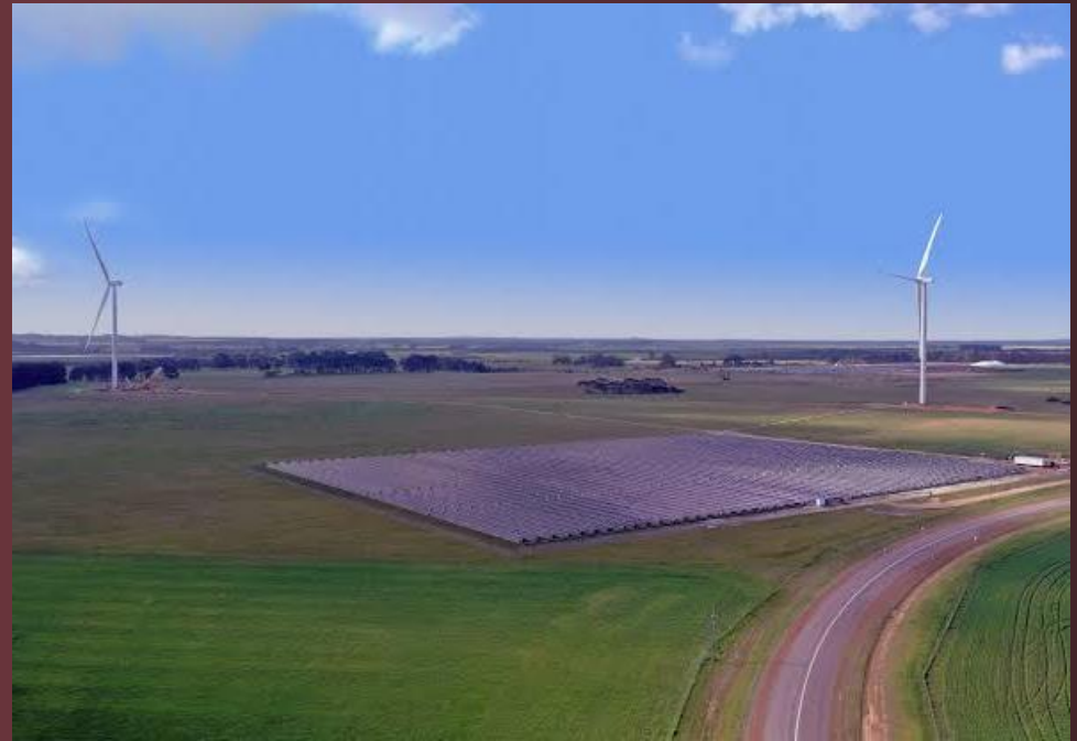
Existing Esperance township 2x 4.5Mw Wind Turbines and 4MW Solar Farm
