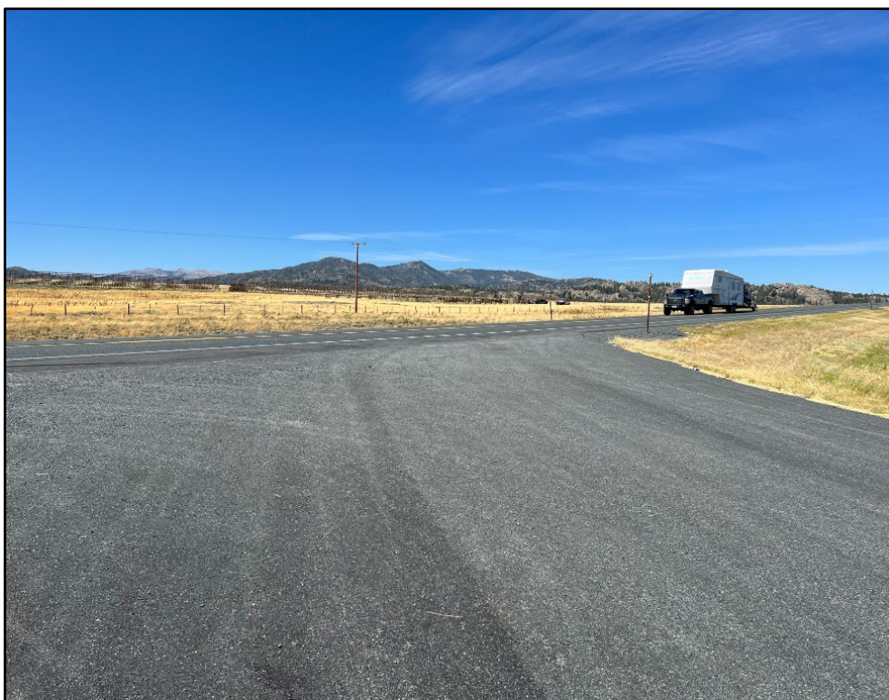
Figure 5. Highway WY-28 which intersects the Project area providing excellent access. Wind River Range in background.
