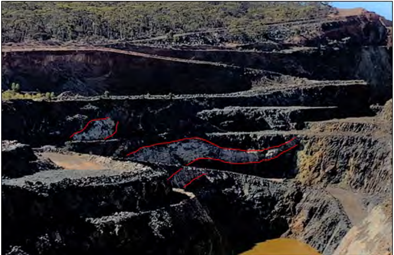
Figure 26: Mt Henry Pit looking north showing flat lying pegmatite exposure (red outline) Source: KAL
