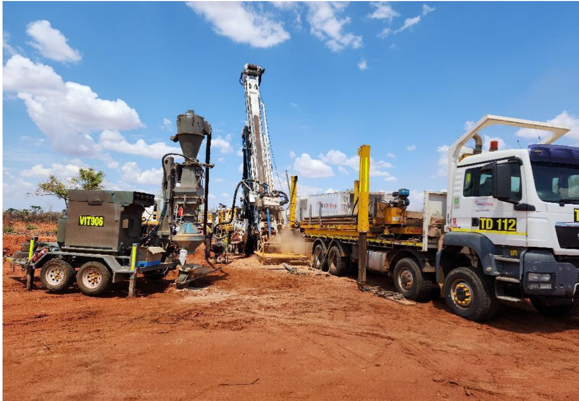
Figure 1: Tulla Drilling Rig 6 operating on-site.
