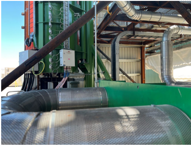
Reactor, furnace, heat exchangers and high temperature piping ready for commissioning at the CDP.
