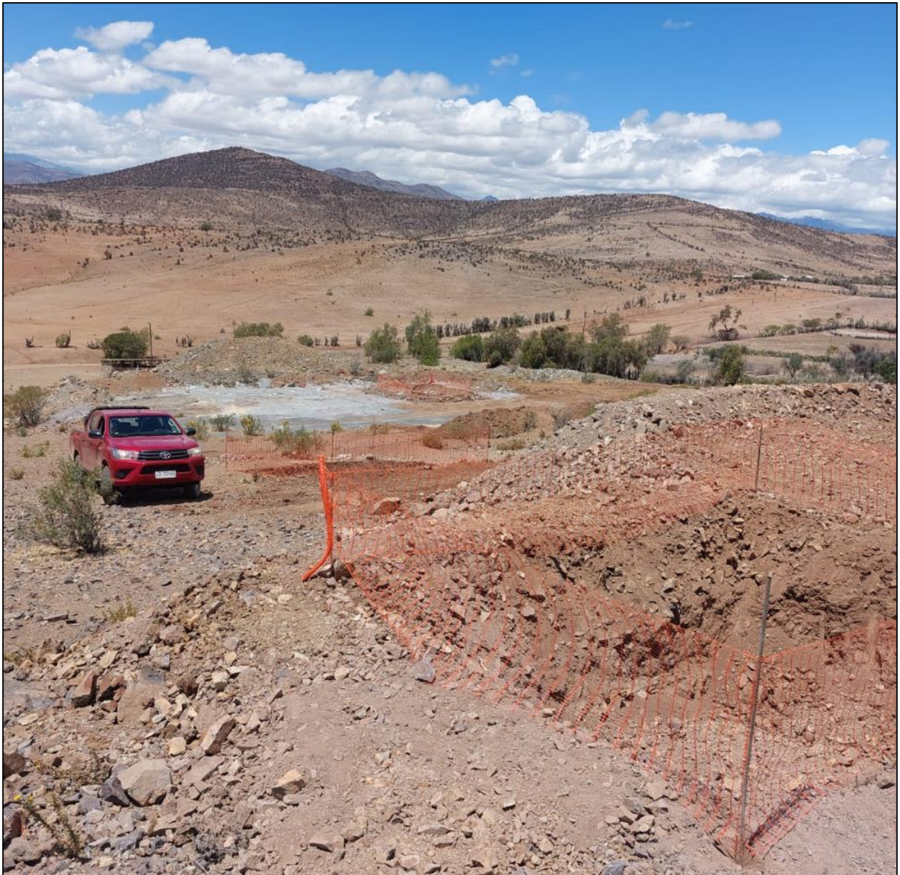
Figure 4: Drill pads constructed at the high priority El Quillay drill target.
