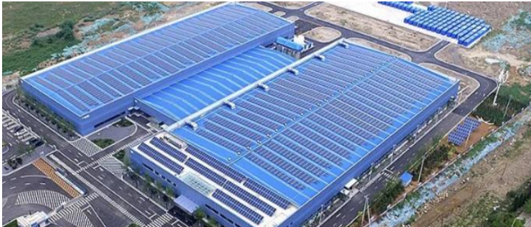
China builds world's largest lithium-free battery - an 800 MWh vanadium redox flow battery.
