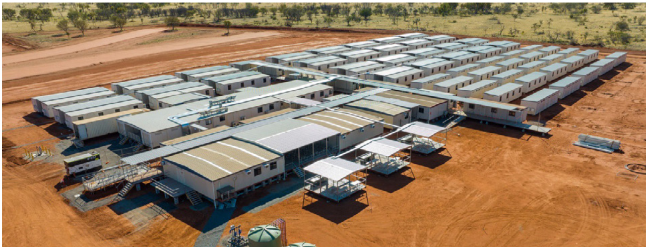
Figure 3. An aerial view of stages 1 and 2 of the Nolans Project construction camp, with capacity to house up to 200 rooms.
