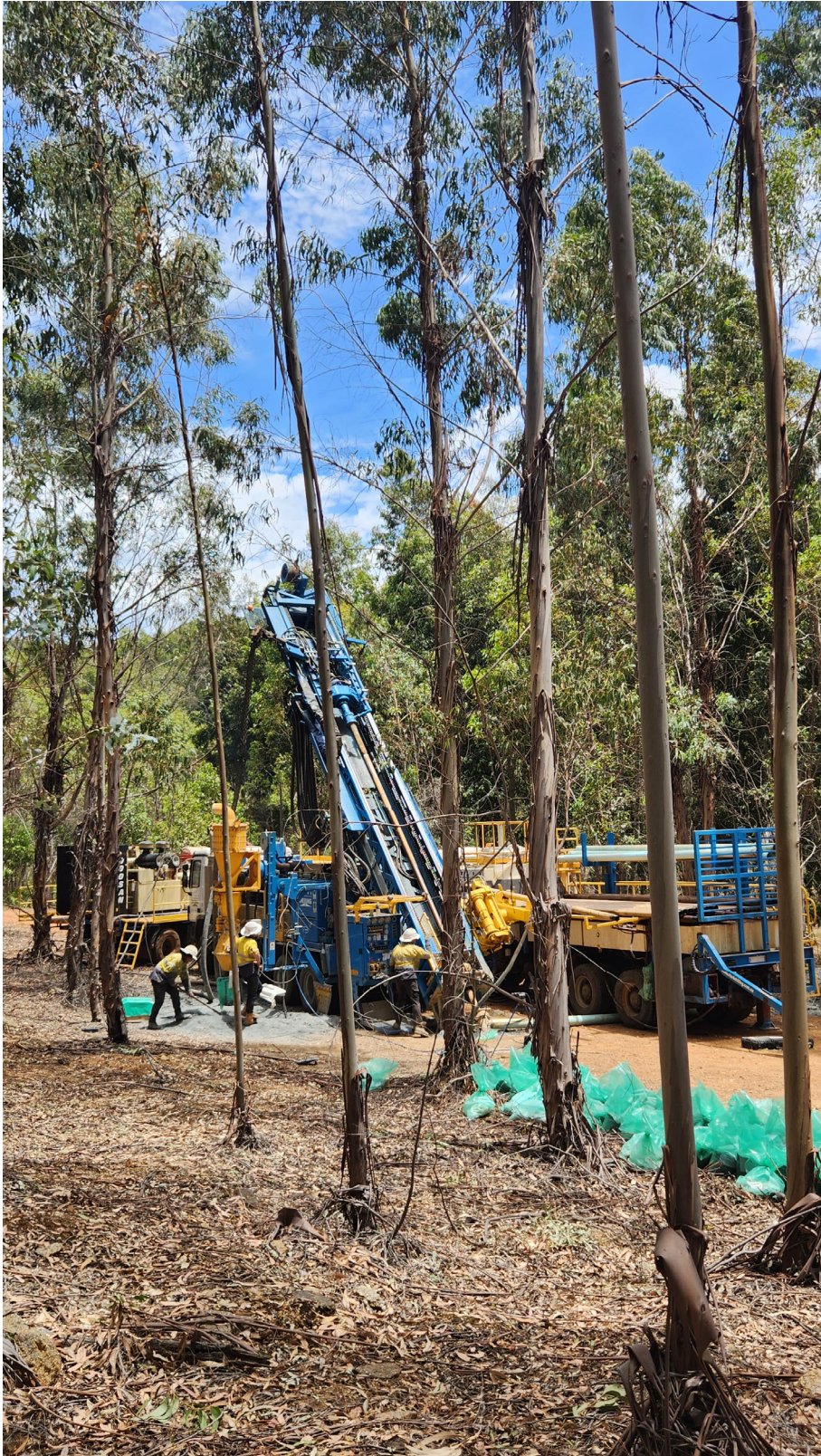
Figure 3: RC Rig on location at the Cobra Prospect.
