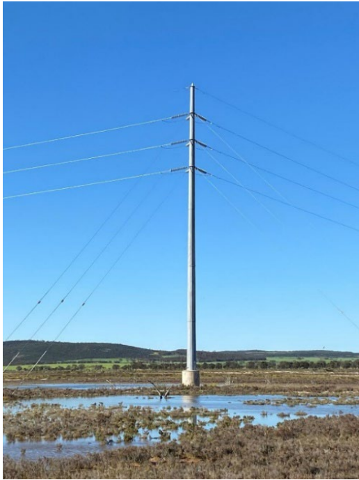
Figure 2: Existing 132kV Moora-to-Wongan Hills powerline (currently energised to 33kV) adjacent to the Project.
