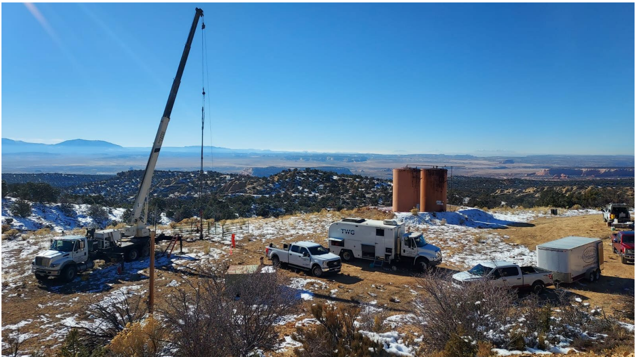
Figure 1: Wireline unit conducting sampling operations at Big Indian #1
