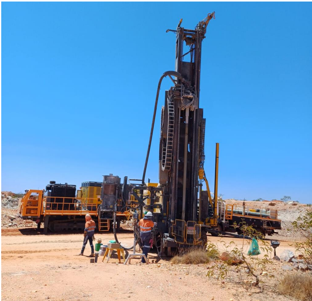
Figure 1: RC Drilling at Pippingarra Quarry Project
