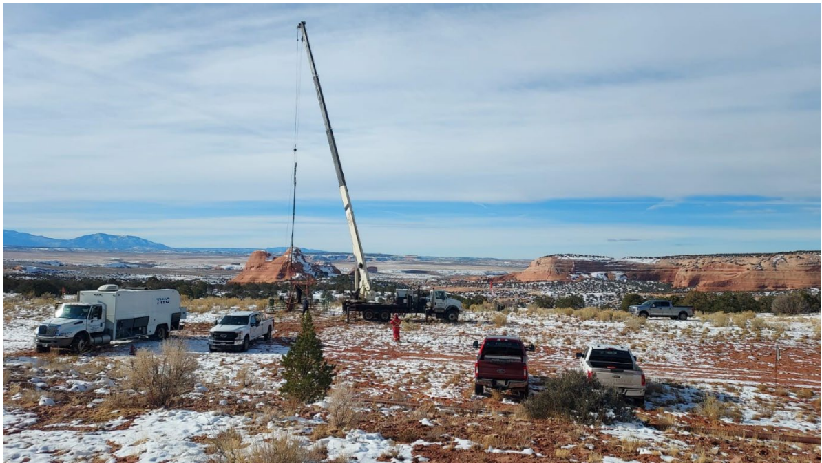
Figure 2: Wireline Sampling at the Hook n Ladder Fed 15-25 well
