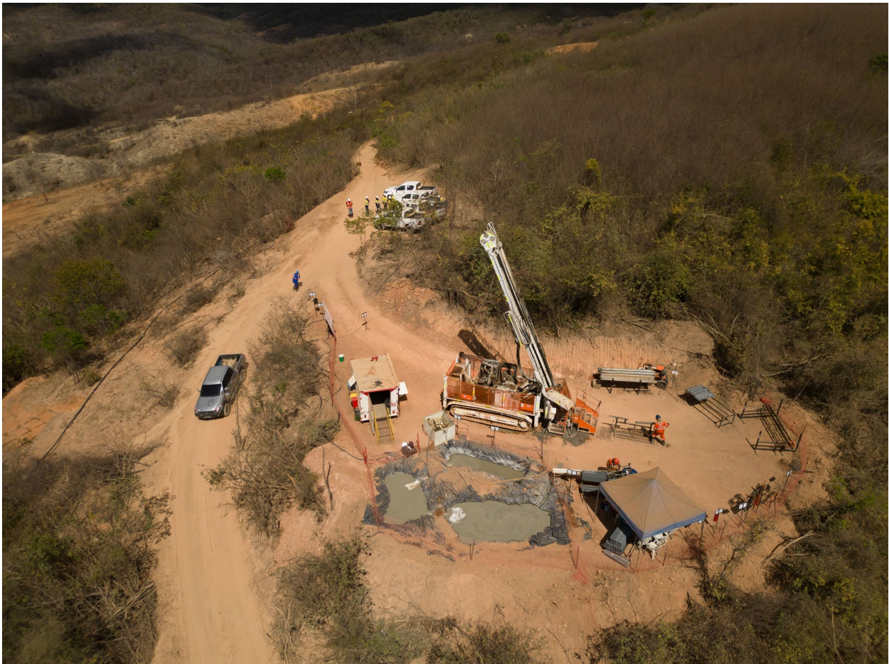
Figure 8: Diamond drill rig on site at Colina Deposit.
