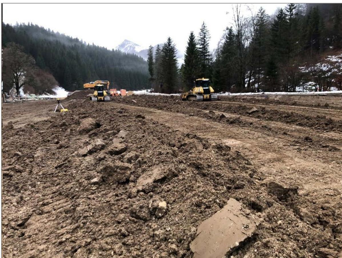
**Well construction operations clearing top soil before installation of foundation material for drilling at the Welchau-1 well site**
