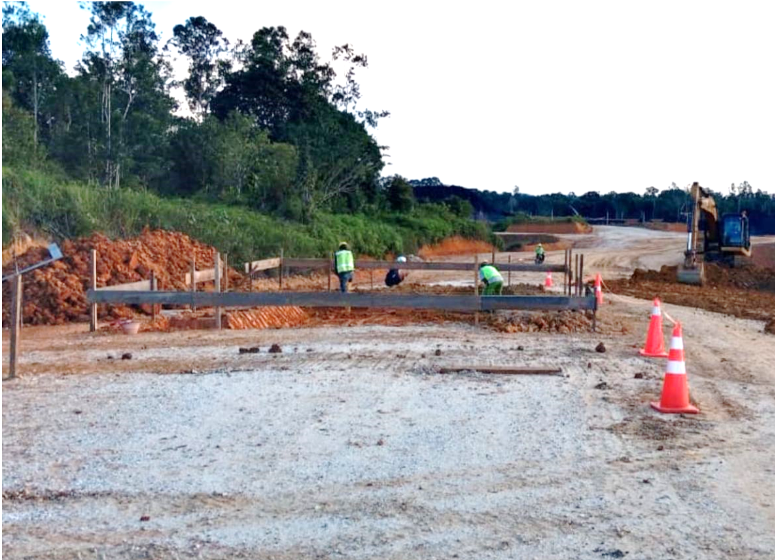
Weighbridge civil works at the Batu Tuhup Jetty
