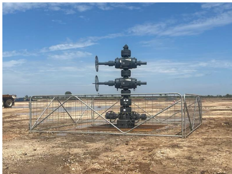
Wellhead installed at Daydream-2
