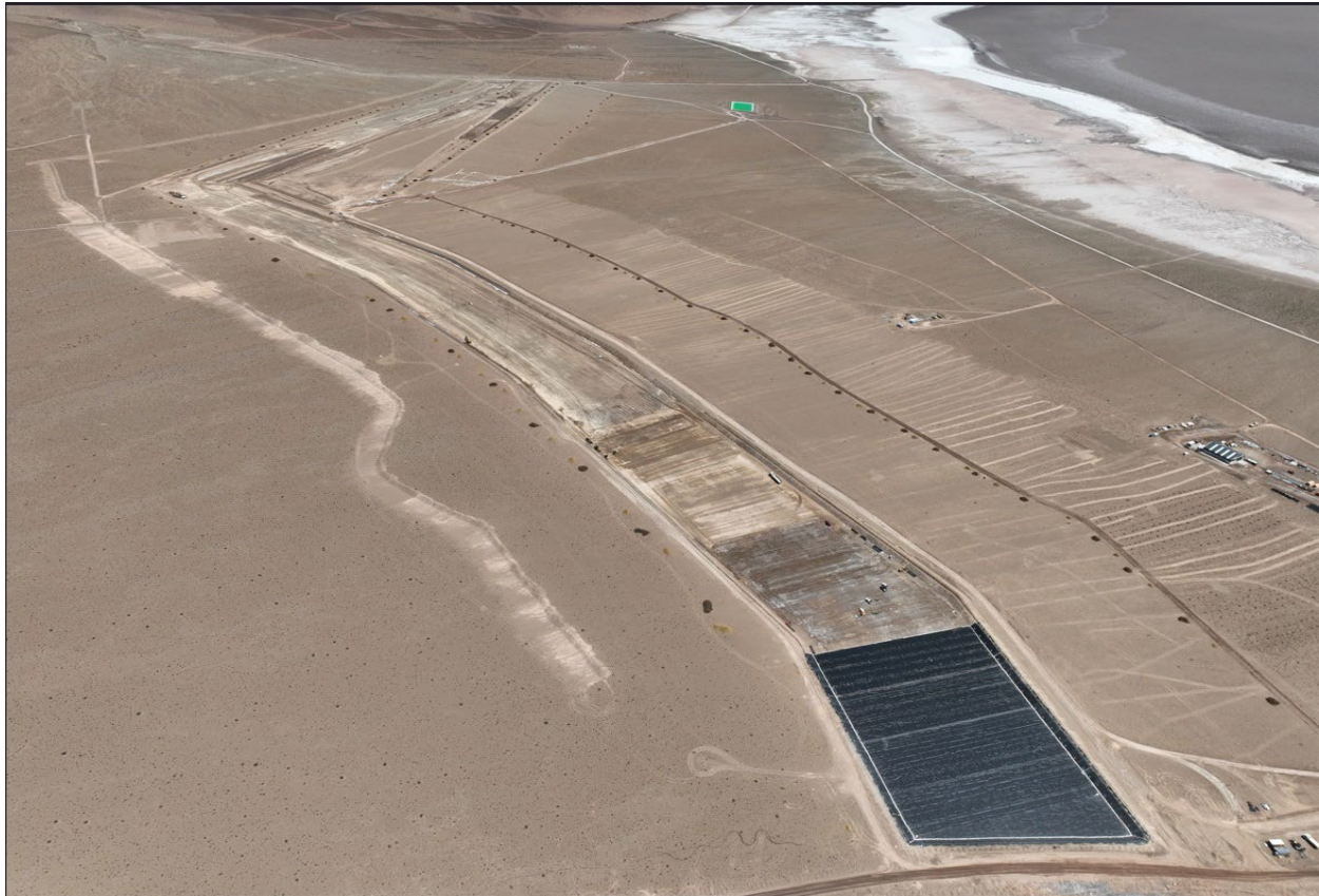
Overall progression of liner installation on Pond 1
