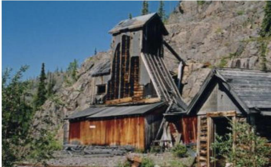
Photo 2 Contact Lake Mine headframe, July 2005.
