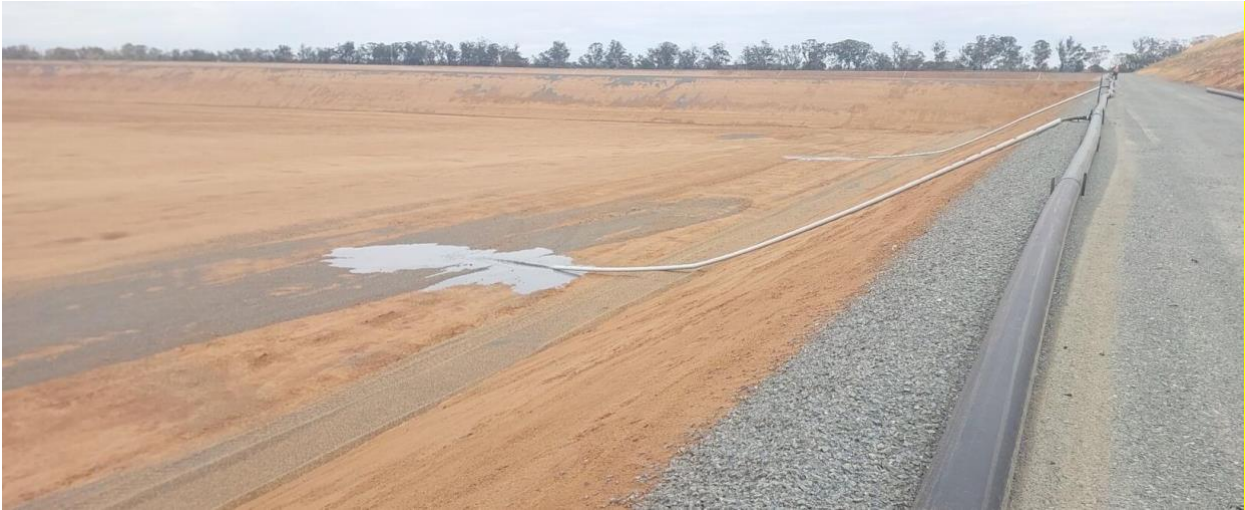
First tailings deposition in RSF2 Cell 1
