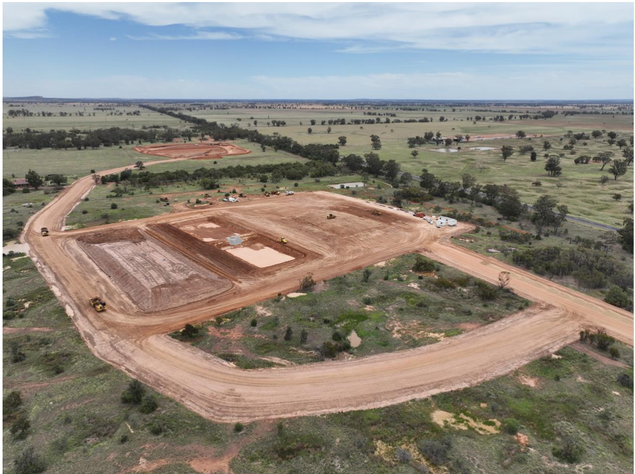
Paste plant pad and earthworks
