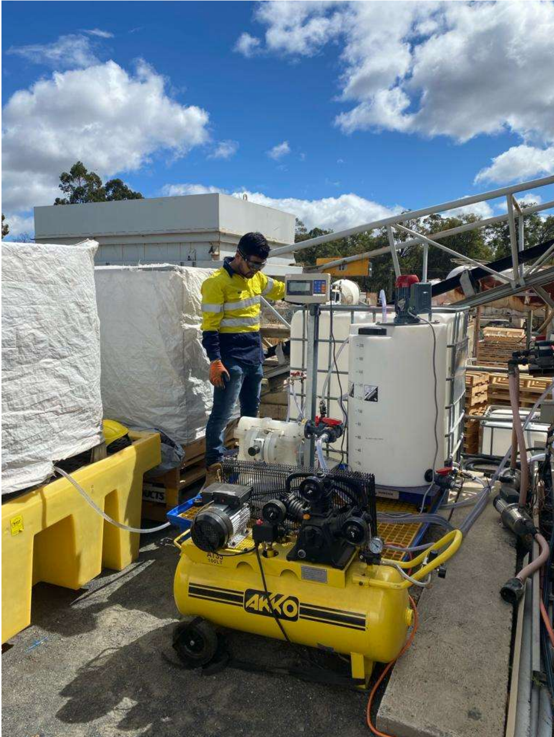
Figure 1 - Geopolymer Pilot Batching Plant
