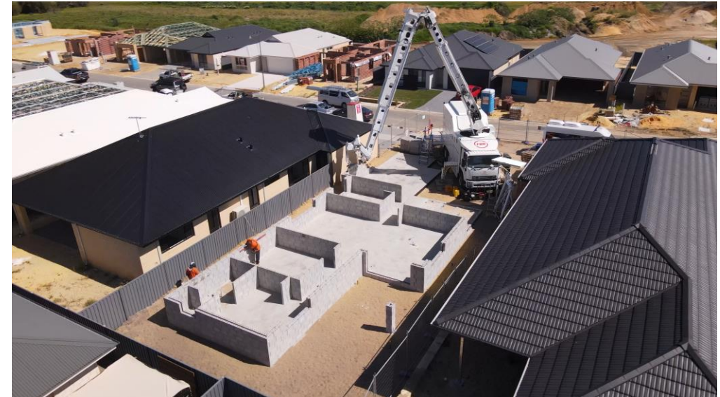
Hadrian X ® building a structure in Wellard, generating zero on-site waste
