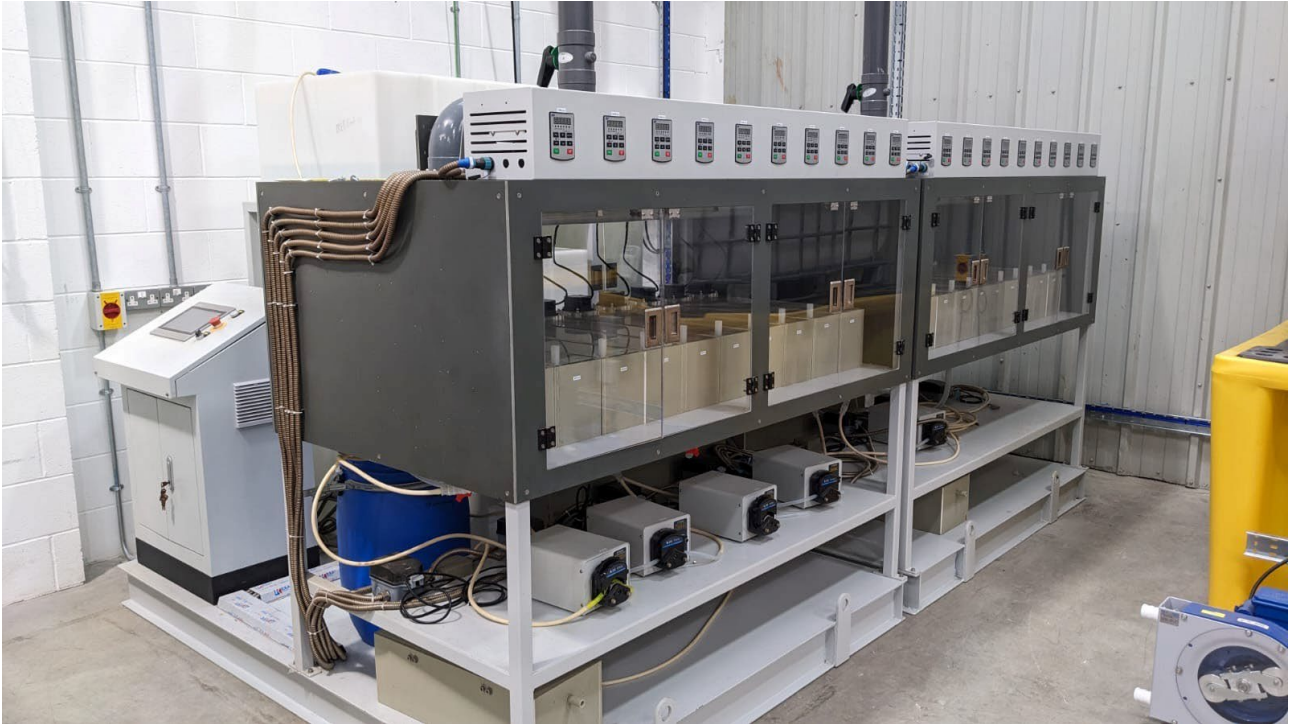
Figure 6: Separation circuit mixer-settlers post water commissioning ready to receive feed stream.
