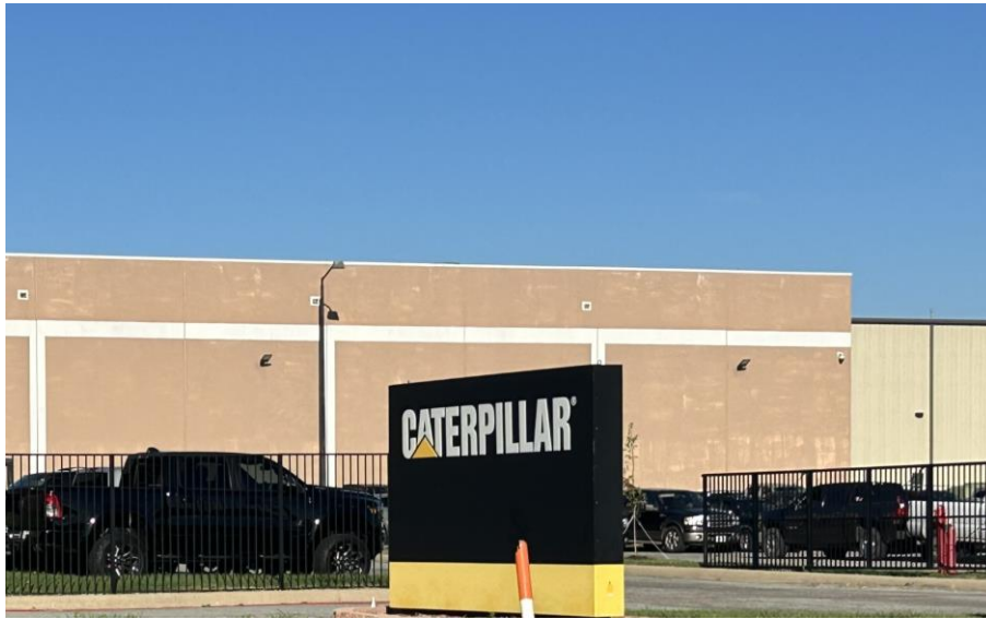
Figure 7 Caterpillar Production Facility - Denison, Texas
