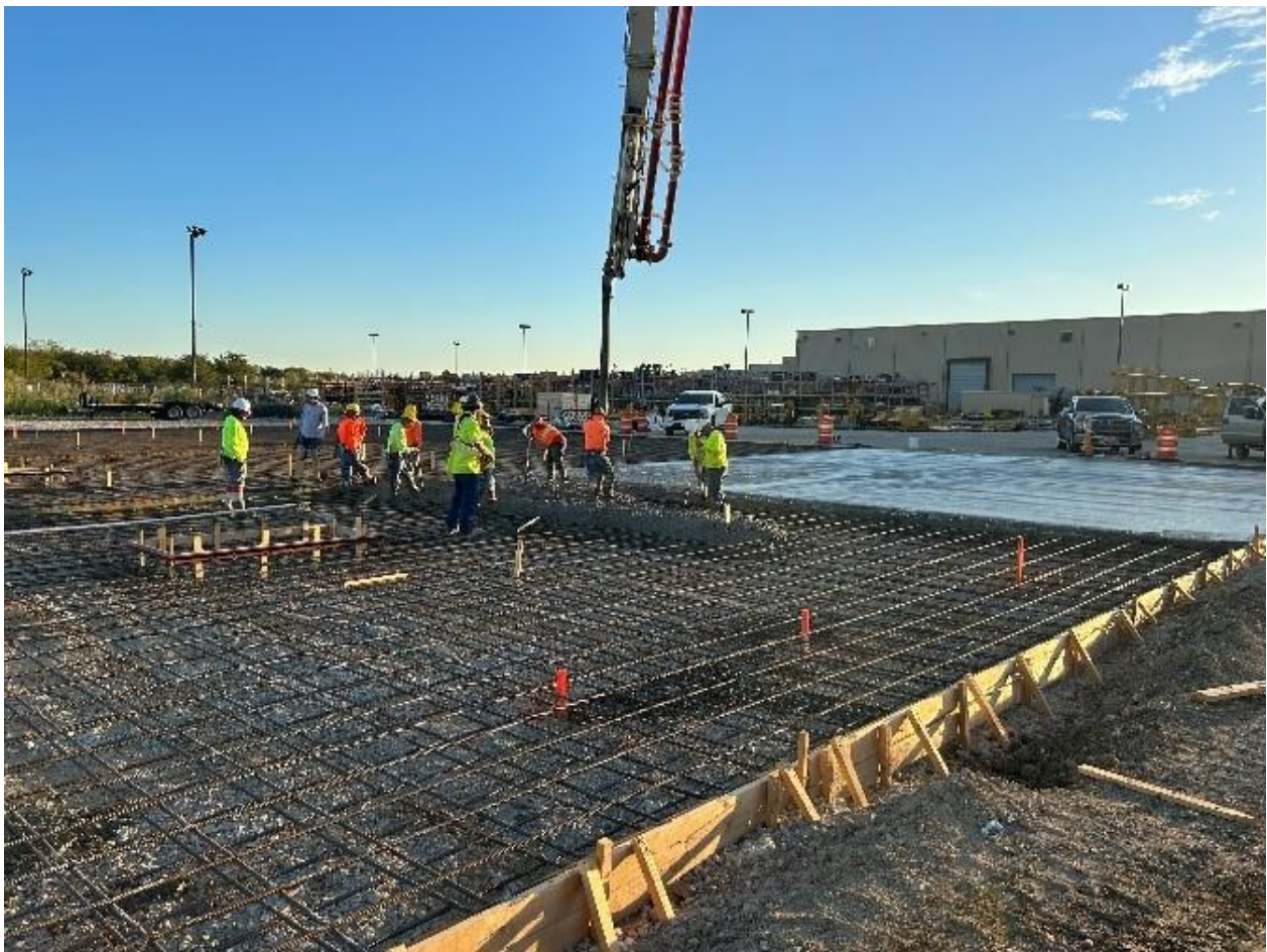
Figure 8. Caterpillar Drill Test Slab - concrete test slab being installed.
