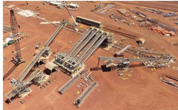
Ken's Bore crushing plant works
