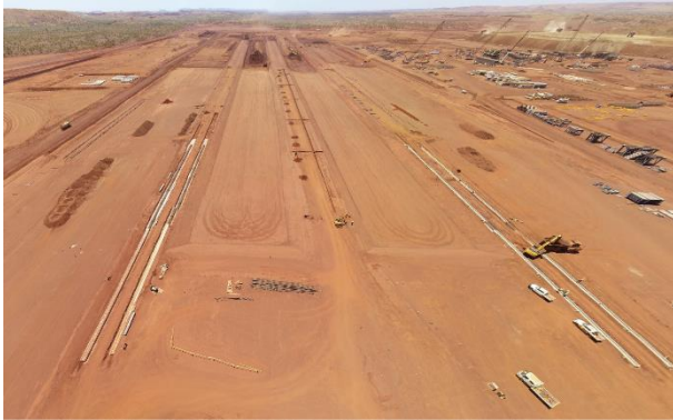
Stacker works and stockyard earthworks
