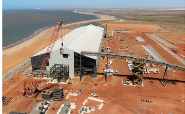
Port of Ashburton ore storage shed
