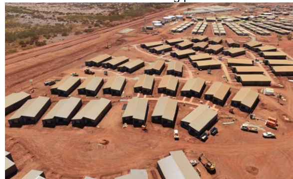
Resort installation progressing
