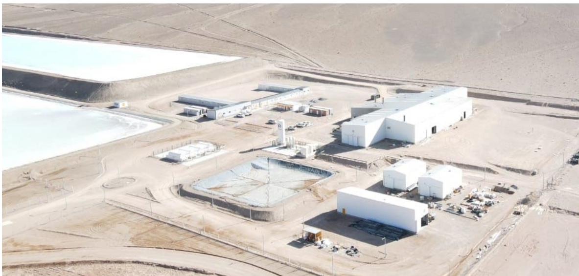
Figure 1. Rincon Lithium Project – 2,000tpa Operations
