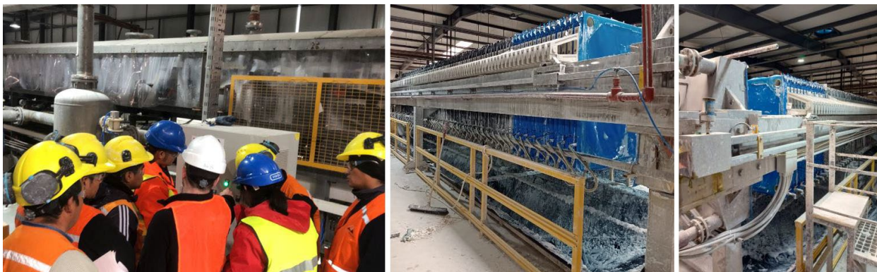
Figures 2-4. Rincon Lithium Project – 2,000tpa Operations
