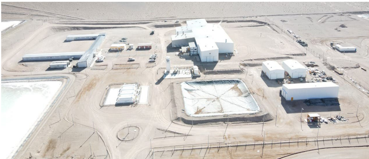
Figure 6. Rincon Lithium Project – 2,000tpa Operations
