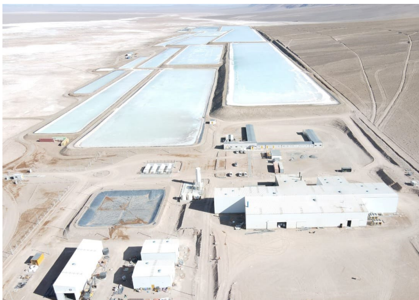
Figure 5. Rincon Lithium Project – 2,000tpa Operations
