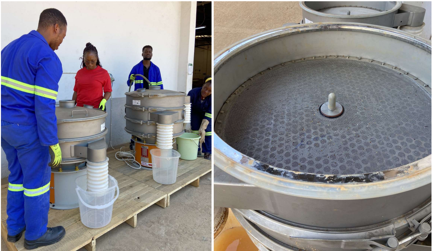
Figure 3. Installation of the new Kwatani 30-inch single-deck and double-deck vibrating separators for sizing and de-sliming bulk samples at the Company's Malawi laboratory and metallurgical facility
