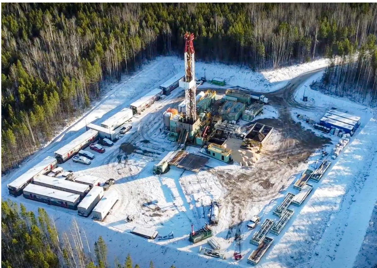
Figure 2. Gryphon Wapiti well site with drill rig.
