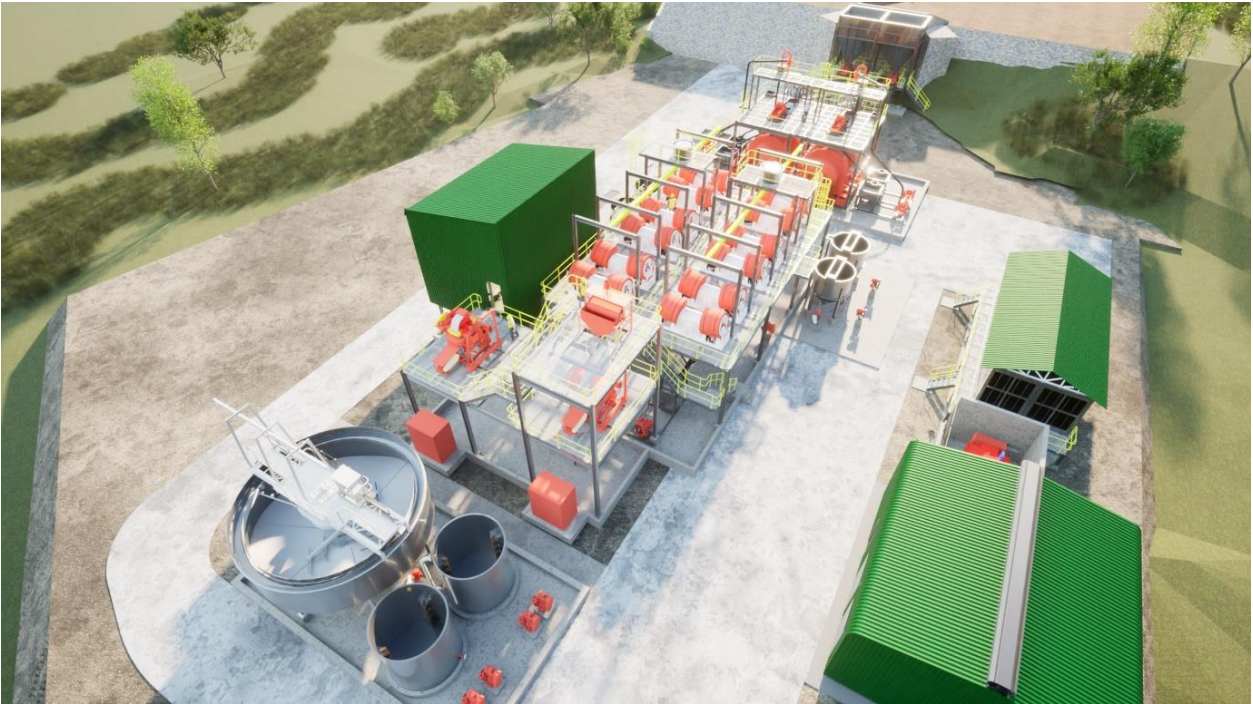
Image 5: Elevated view of the recovery circuit and tailings thickener.
