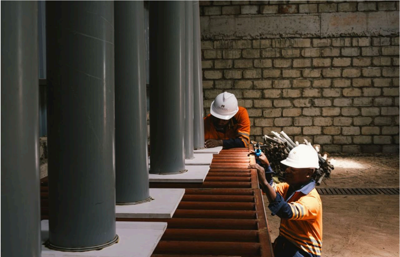
Figure 5: Inspection of constructed desorption columns.
