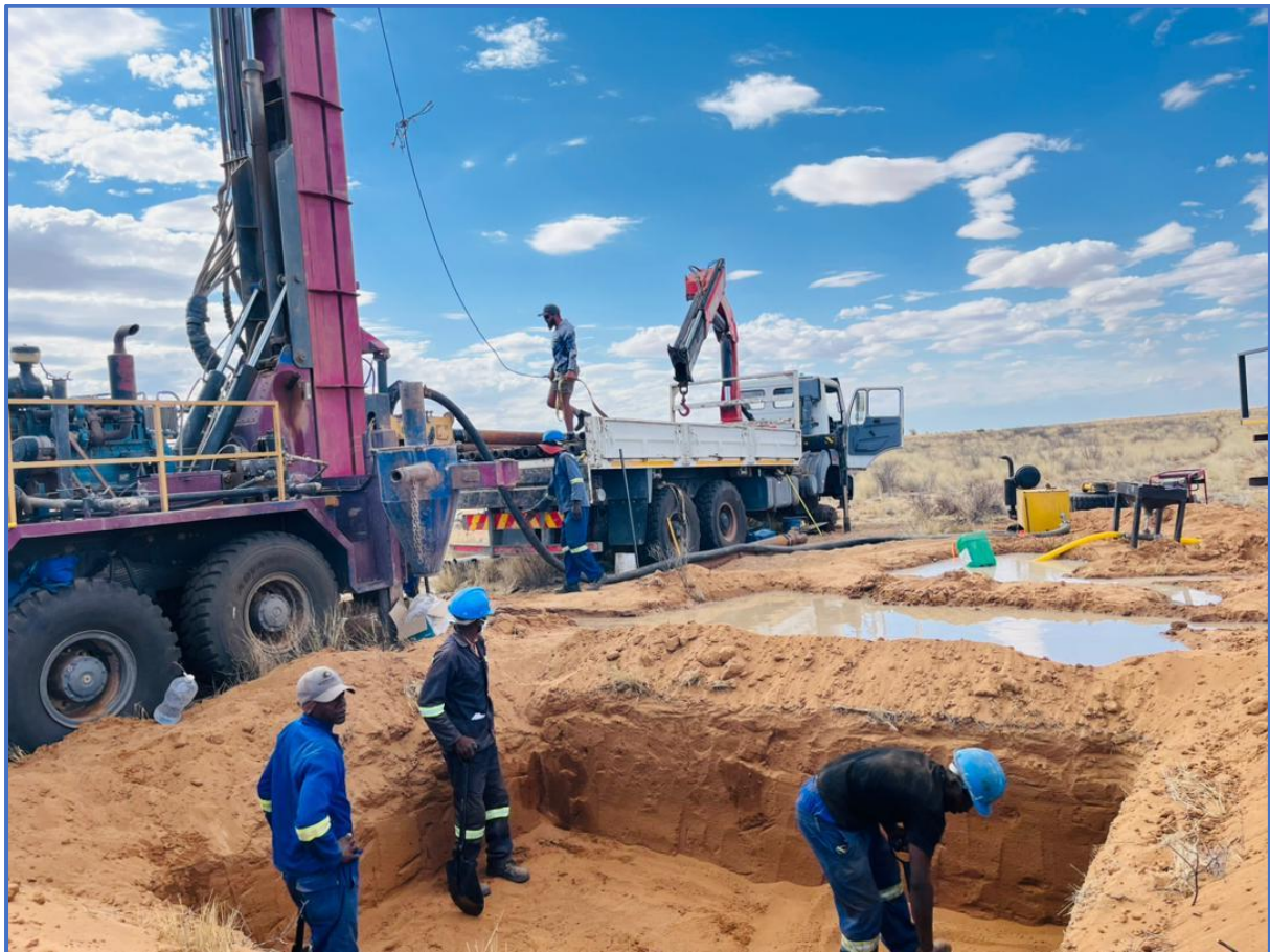
Figure 4: Photo of drilling operations underway 1
