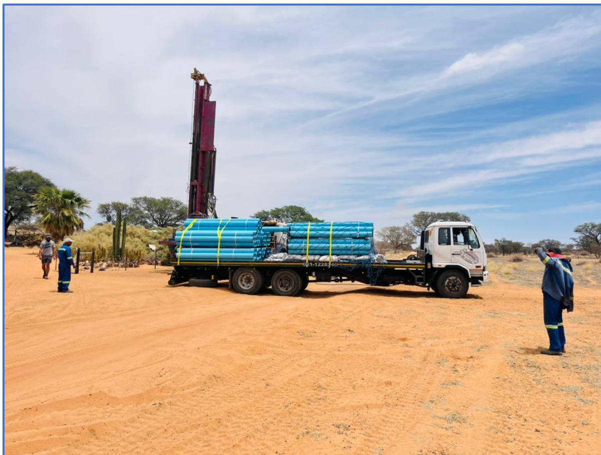
Figure 5: Photo of special casing being delivered 1
