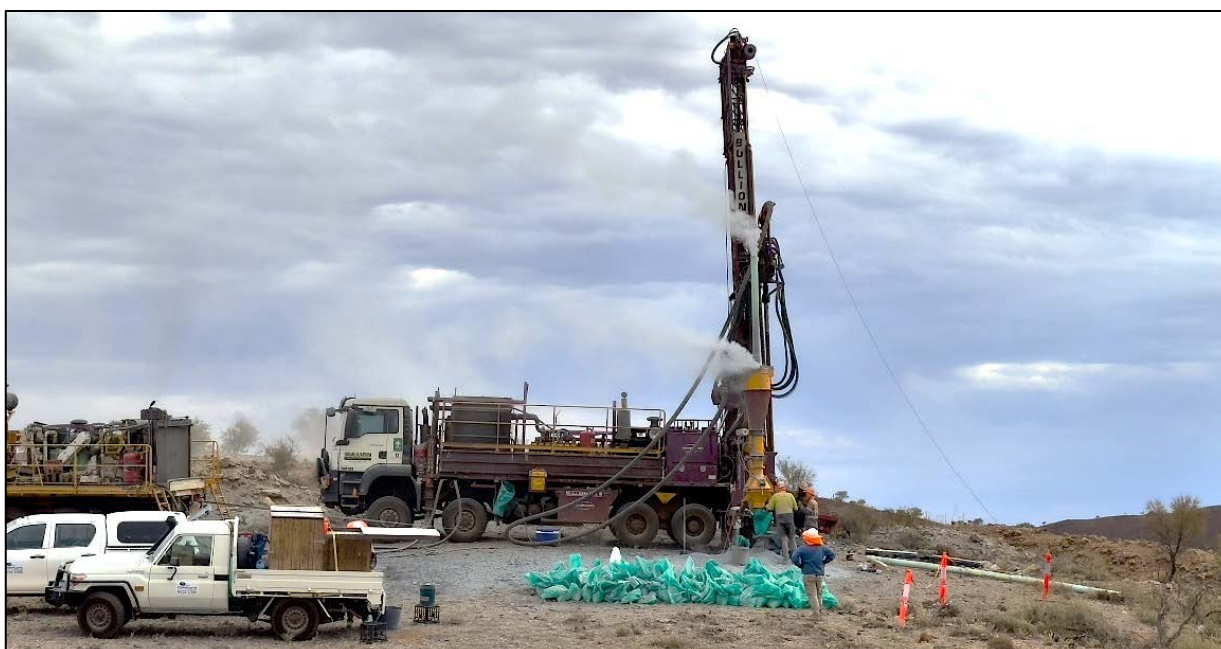
Figure 2 Photograph of drilling TRD001 at the Trident Lithium Project
