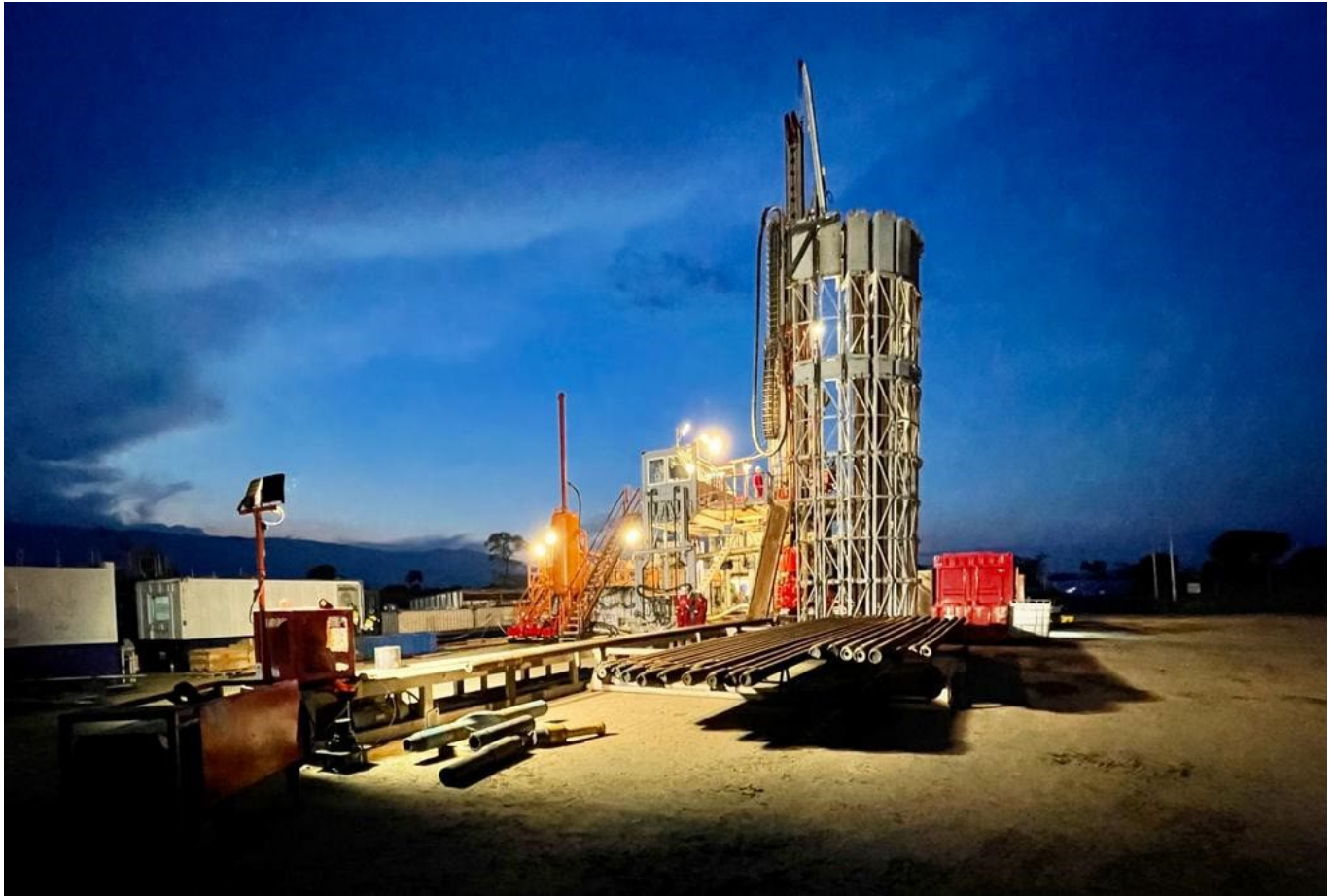
Figure 3. Drilling the Mbelele-1 well at the North Rukwa Project.
