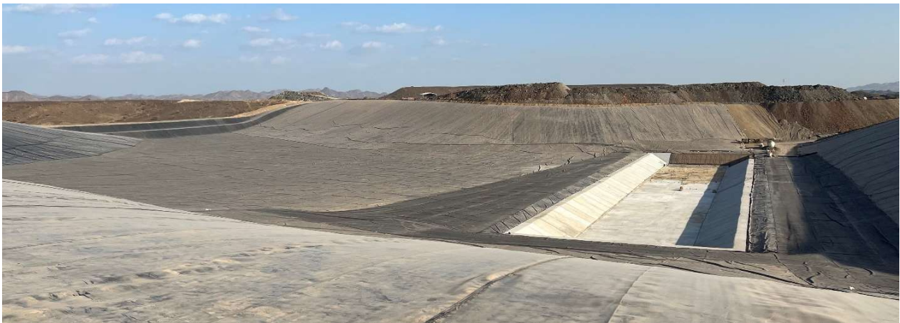
Image: Dry Processed Tailings Storage Facility
