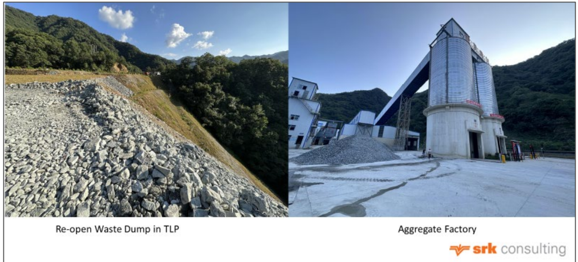
Figure 5-25: Waste dump in TLP and aggregate factory typical shrinkage stoping method
