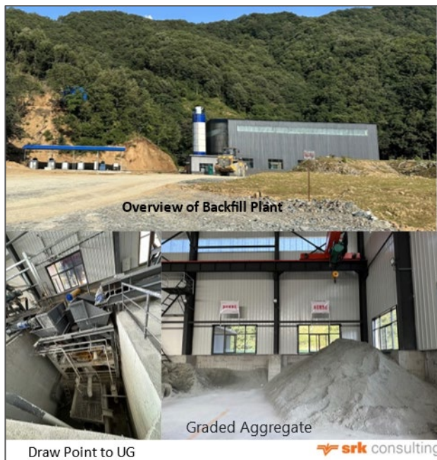
Figure 5-23: Backfill plant at LMW
