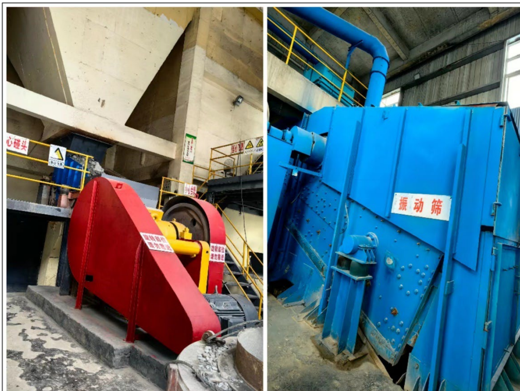
Figure 6-1: The crushing plant as observed during the site visit
