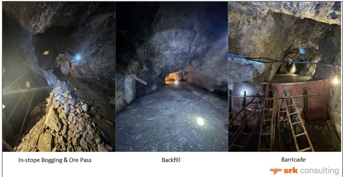
Figure 6-11: Operation of cut and fill stoping
