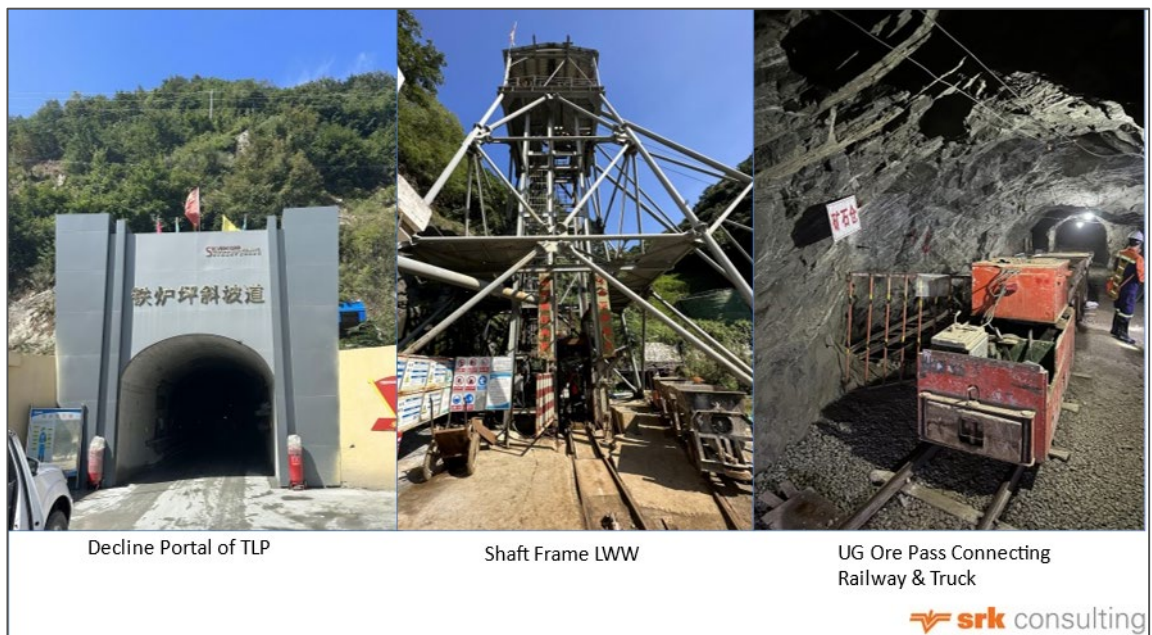
Figure 5-18: Underground access and level drive at the TLP and LMW mines
