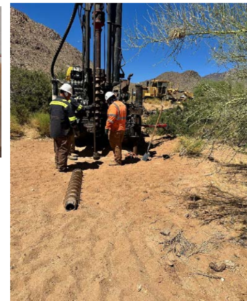
Surface Geotechnical Investigation – Cascade Drilling
