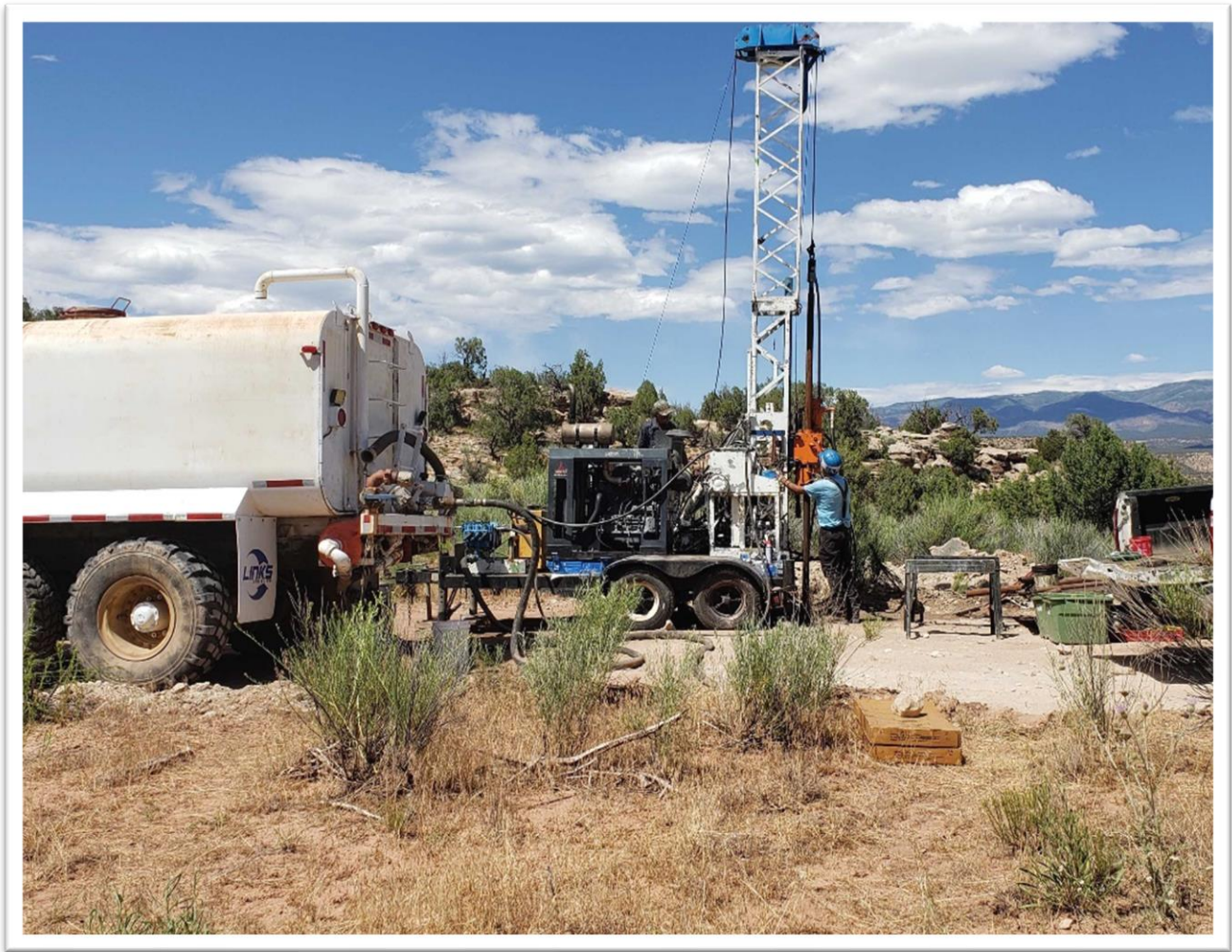
Figure 2 – Drill rig on site – REX Project
