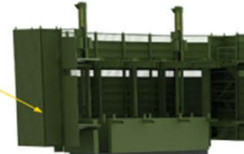
The system climbs with electric ball screw jacks that are computer controlled
