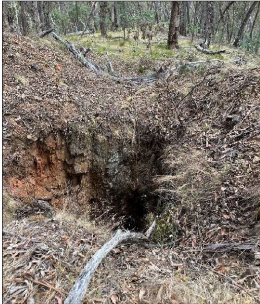
Figure 1 – Vertical shaft/stopes. Located at 710894E, 6259083N.
