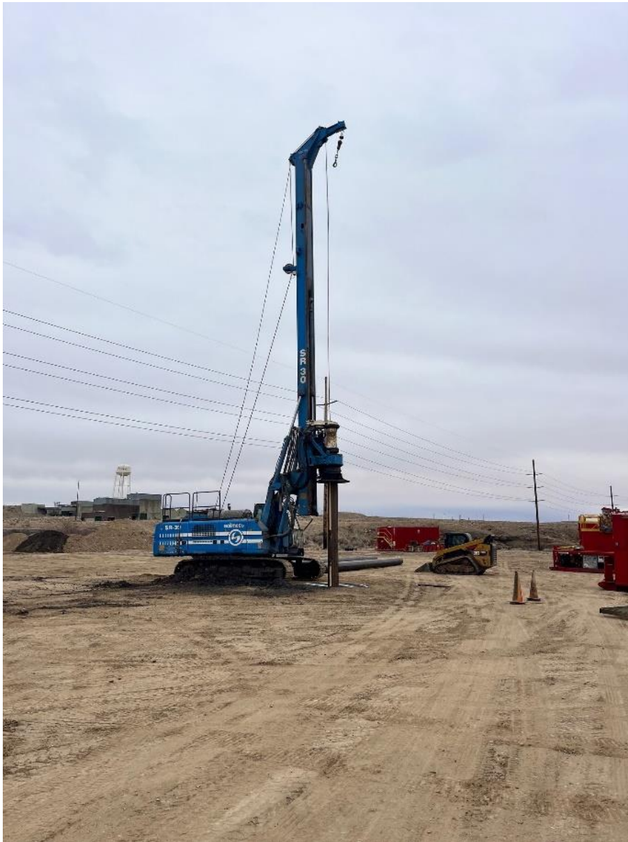
Figure 1: The drill rig setup at the Bosydaba#1 well site.
