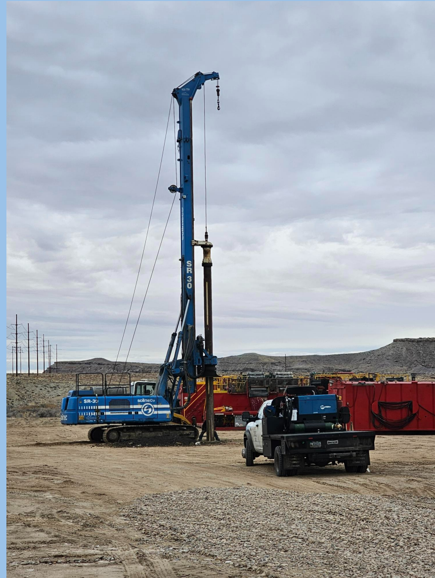
Photo showing the drilling rig at the Green River property
