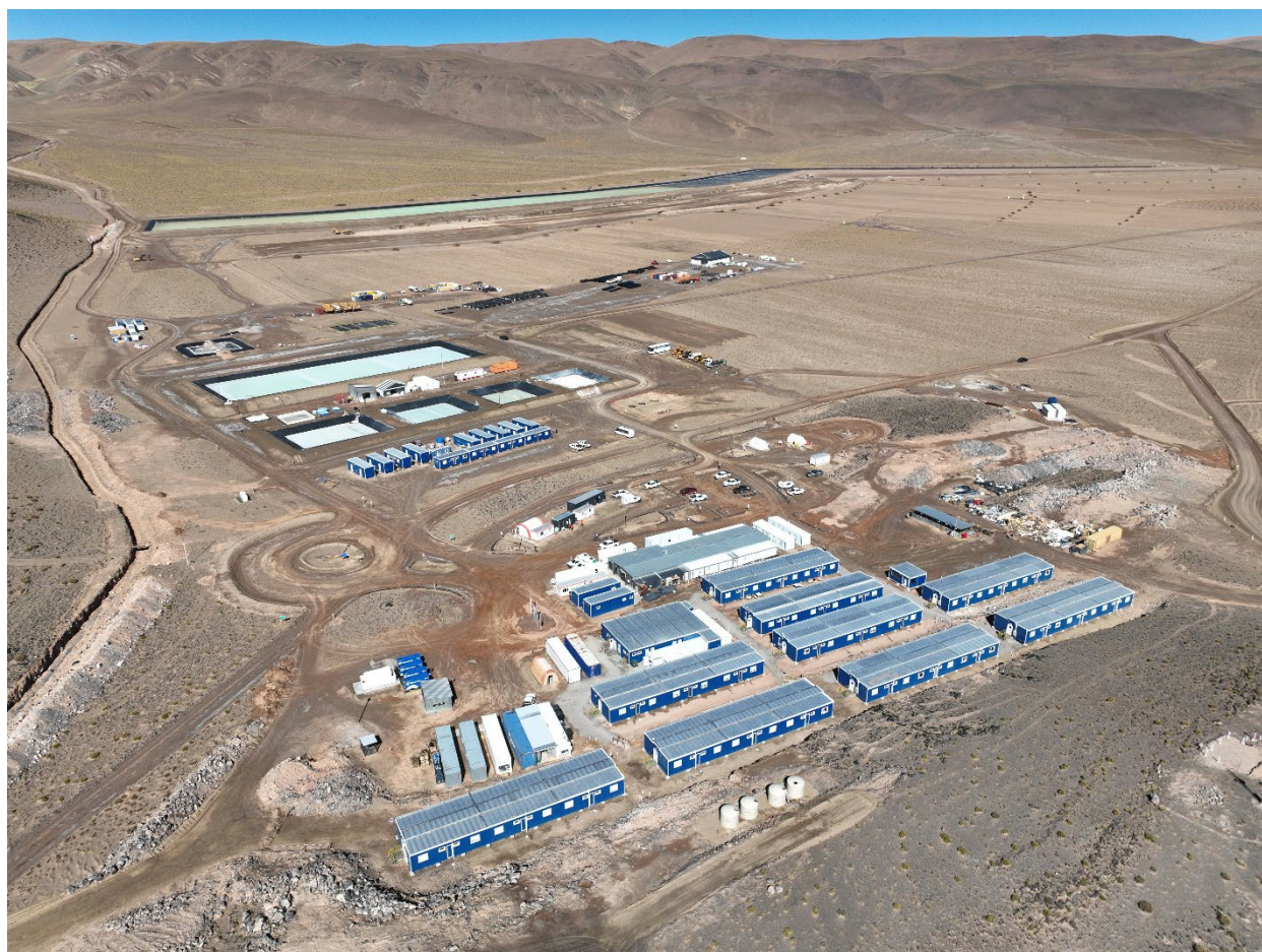
Construction progress at HMW (February 2024)
