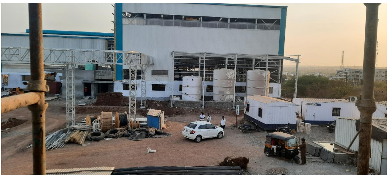
Figure 1- the main production structure on site
