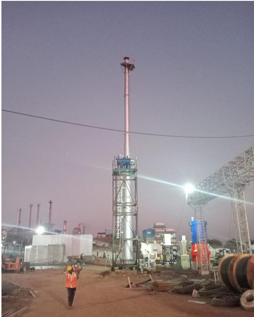
Figure 5 – Substantial infrastructure on site – February 2024
