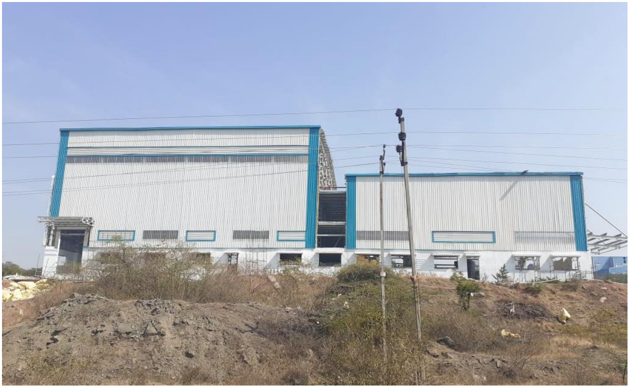
Figure 3 – External Infrastructure during the final week of construction
