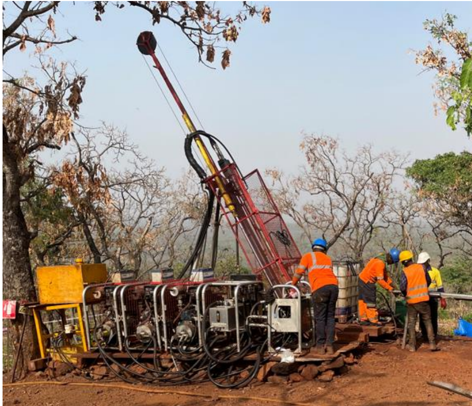
Figure 6: Energold Ranger drill rig completing drill hole DALDDH008 at the Dalabatini prospect
