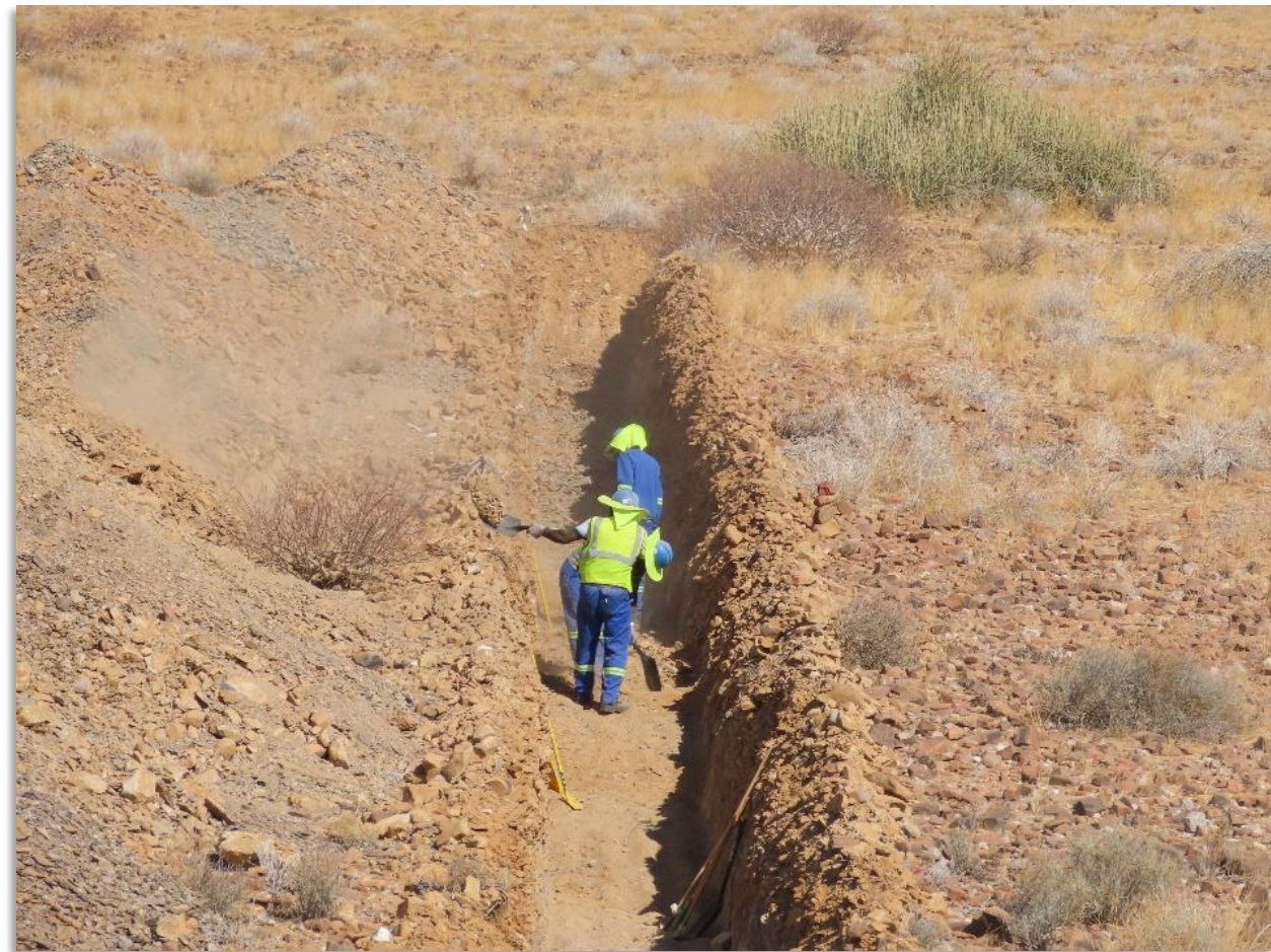
Figure 4: Clearing OP-T19 trench for sampling
