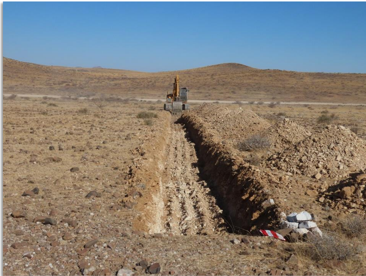
Figure 3: Excavator trenching OP-T7
