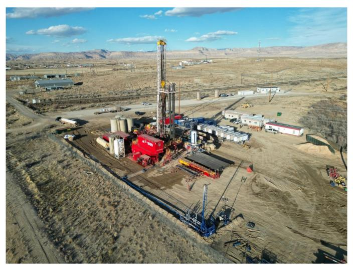
Figure 1: The drill rig setup at the Bosydaba#1 well site with the Sample Demonstration Plant in the background.
