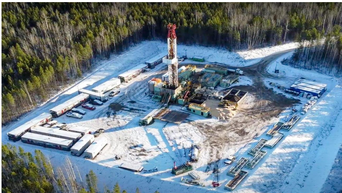
Figure 3. Image of the Gryphon Wapiti well site with drill rig.
