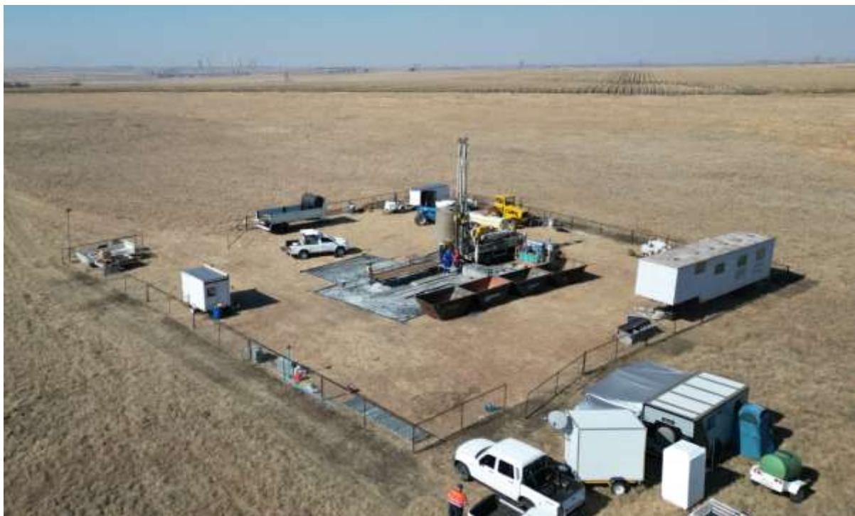
Figure 5 – Location of 272-06C with Sasol's Secunda plant in the background
