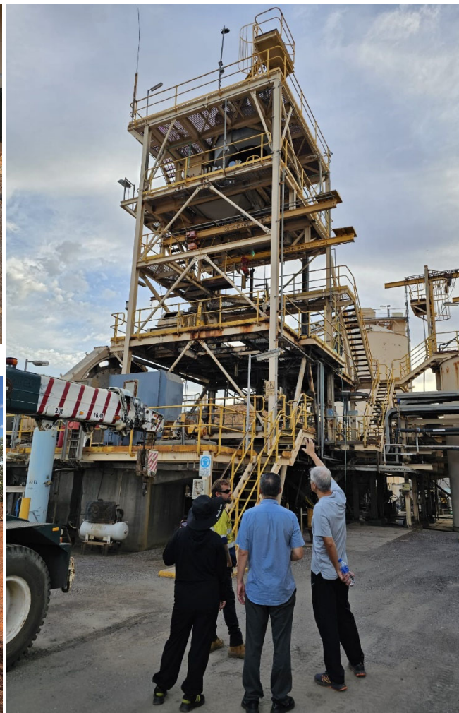
Figure 3: Sundry representatives inspecting refurbishment at Paulsens
